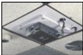
Finished installation of the Dukane Projection System
