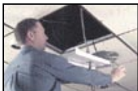
Ceiling mount replaces 2'x2' ceiling tile.
